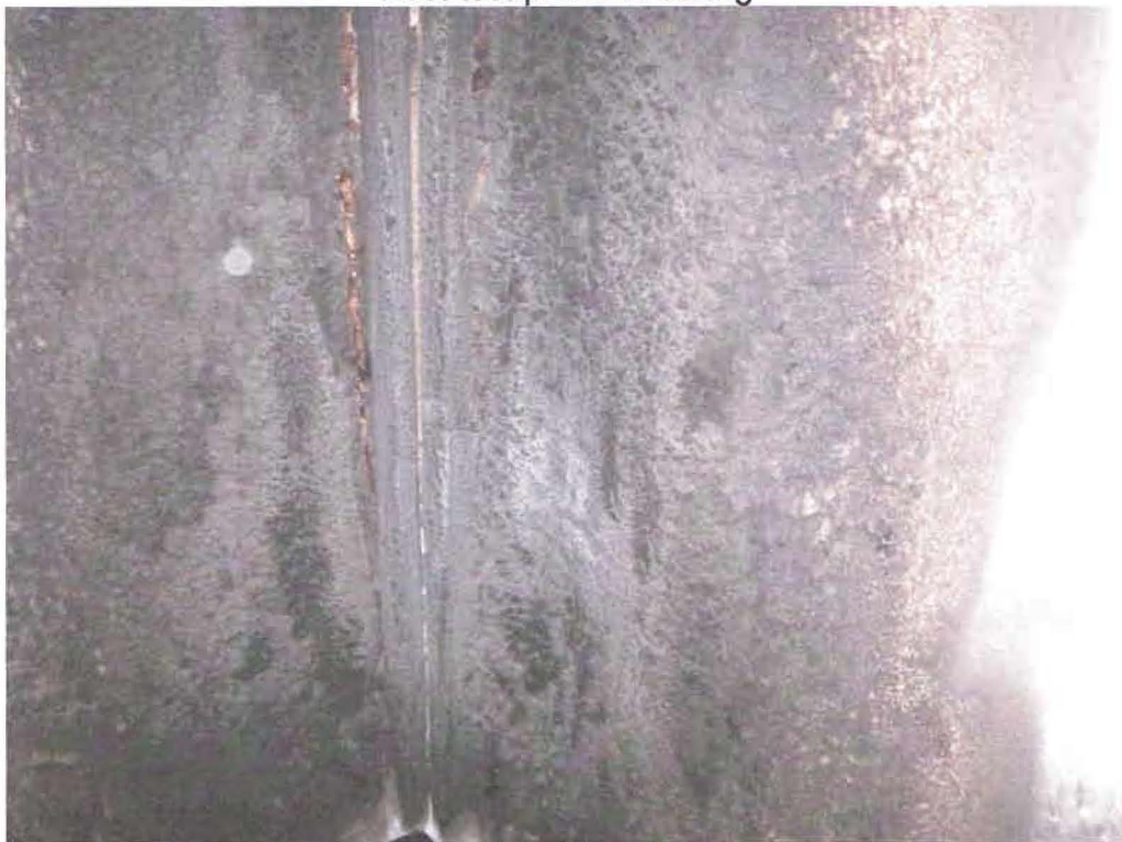
Detail of corner
