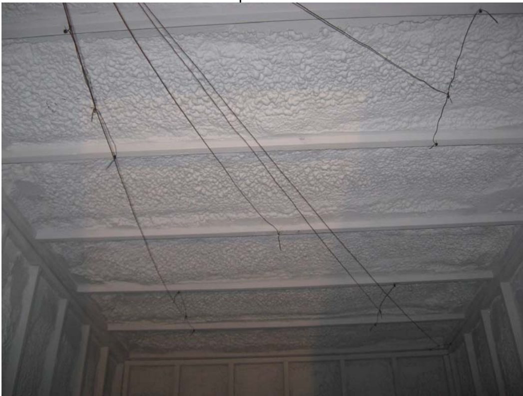
Pre-test photo ceiling
