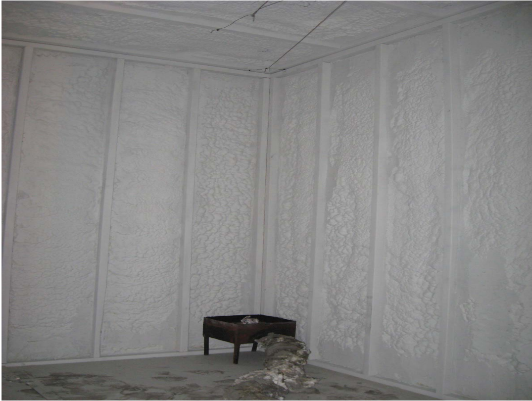
Pre-test photo corner.
