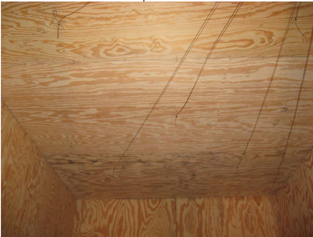
Pre-test photo ceiling
