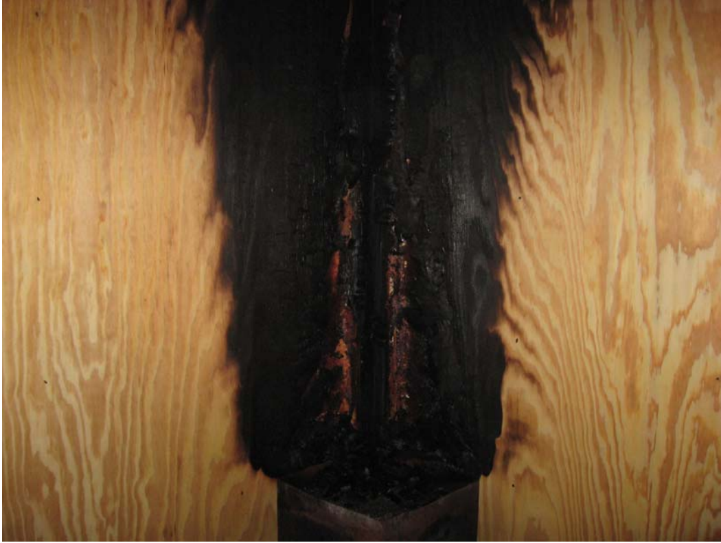
Detail of corner
